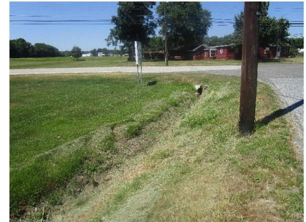
The trench alongside the south side of the road next to the “Canton Baptist Church” sign can be transformed into a rain garden to allow stormwater runoff from the road to infiltrate and reduce contaminant levels more efficiently while providing a habitat for wildlife. A preliminary soil assessment suggests that more soil testing would be required before determining the soil’s suitability for green infrastructure.
