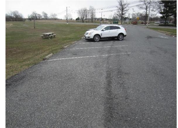
Bioretention systems can be installed in turfgrass at two locations to allow the stormwater runoff from the pavement to infiltrate. The parking spaces east of the pizzeria can be retrofitted with pervious pavement to allow water to penetrate the surface. A preliminary soil assessment suggests that more soil testing would be required before determining the soil's suitability for green infrastructure.
