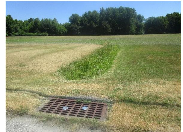
On the east side of the road there exists a bioswale filled with grasses. This can be extended perpendicularly to its current position to create a rain garden, travelling alongside the road to allow stormwater runoff to infiltrate into the ground and reduce contaminant levels. A preliminary soil assessment suggests that more soil testing would be required before determining the soil's suitability for green infrastructure.
